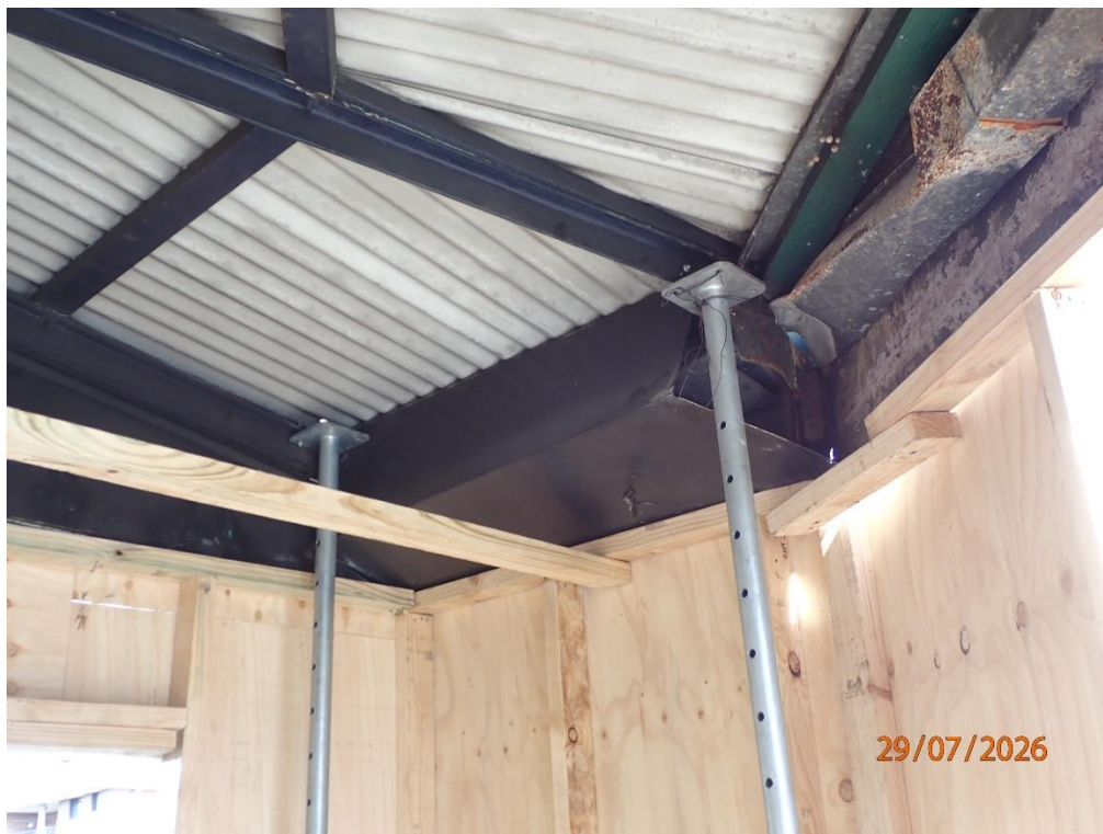
Figure 3. The temporary structures holding the awning in place.
