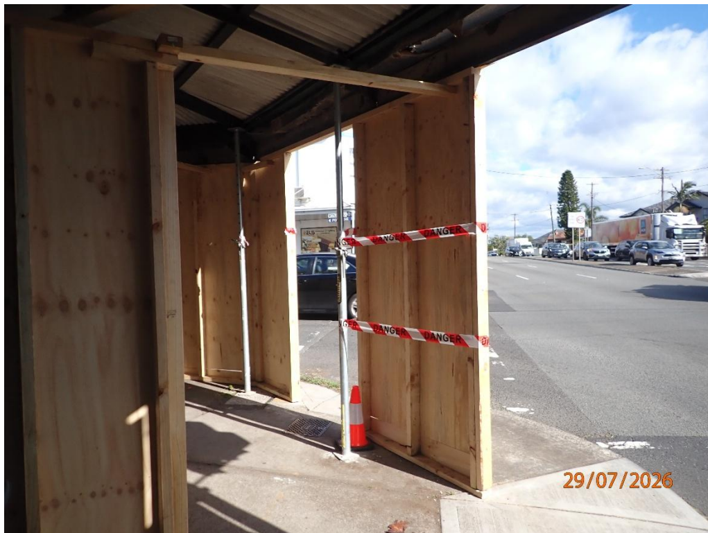
Figure 4. Protective measures to prevent further damage to the awning and to protect pedestrians.
